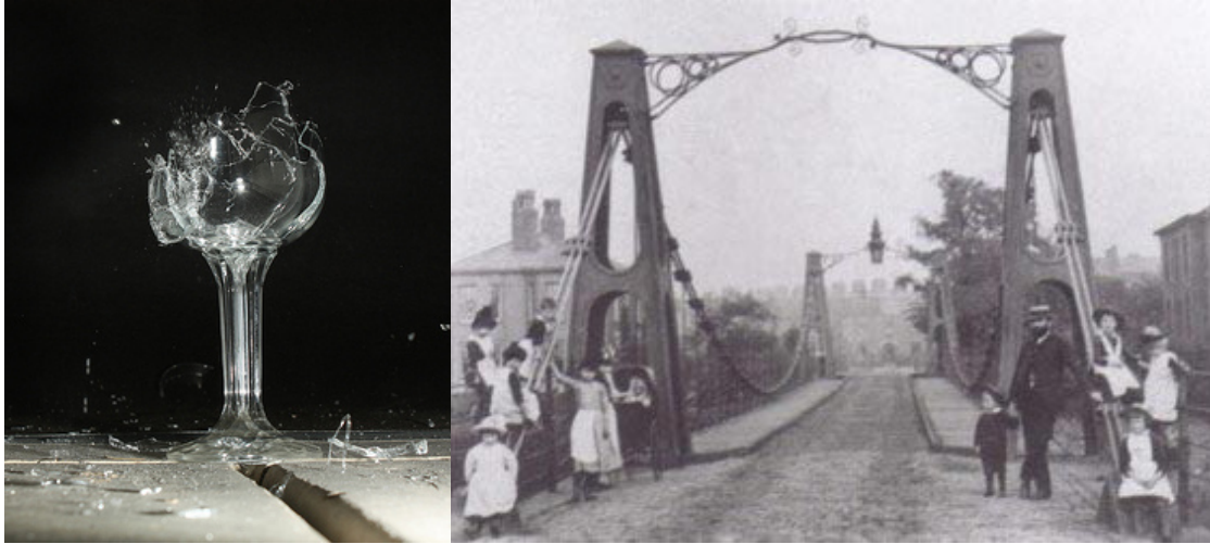
Figure 7.1: ( left ) Resonant vibrations are a common source of fragility in natural objects. Here a glass fails in the presence of an acoustic wave at resonance. ( right ) On a larger scale, structural failure through periodic loading of the Broughton Suspension Bridge caused its collapse in 1831 due to the resonance of the soldiers marching in lockstep [115].
